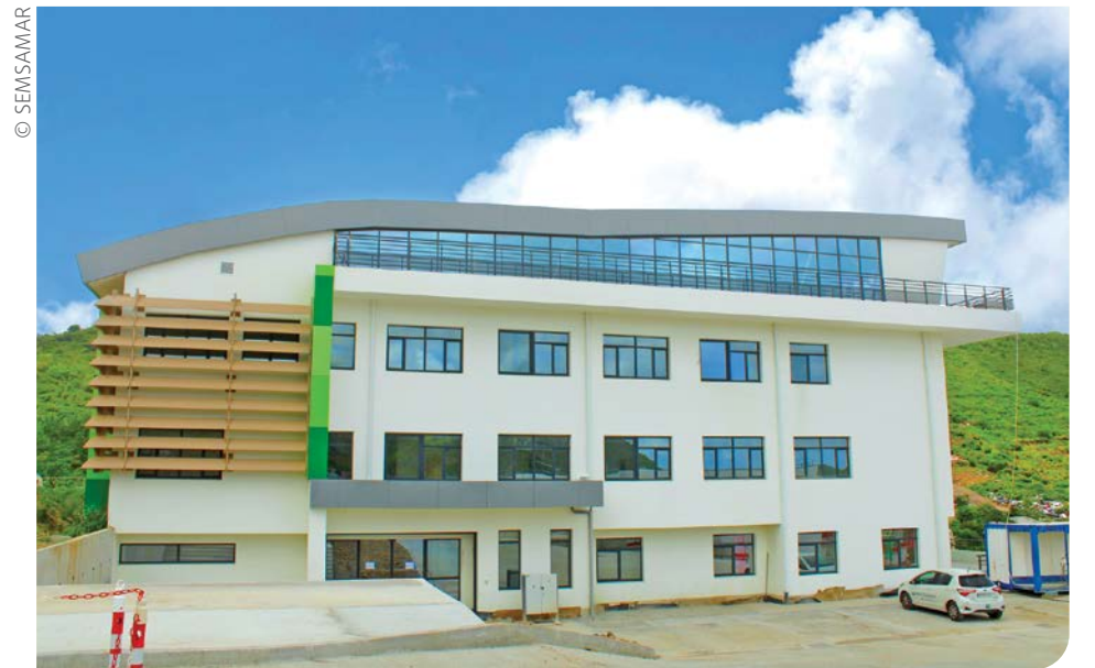
The new Wataki healthcare and rehabilitation unit was developed by Semsamar.
